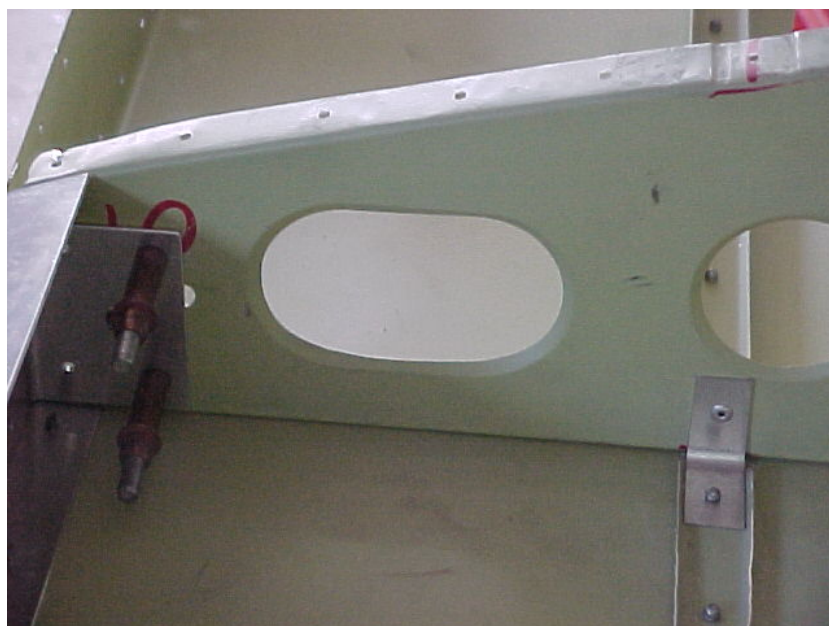
Figure 4.9: Wing tank reinforcement 5.
